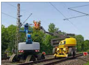
Construction of contact lines
