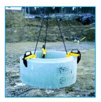
Clamps offer a method of connecting to the load so that it may be presented tight up to a neighbouring component without trapping the lifting equipment.
